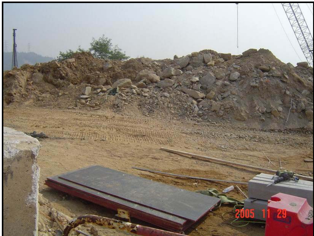
Figure 2 Stockpile at PAFF Construction Site (Photo: Leighton Contractors (Asia) Limited, November 2005)
